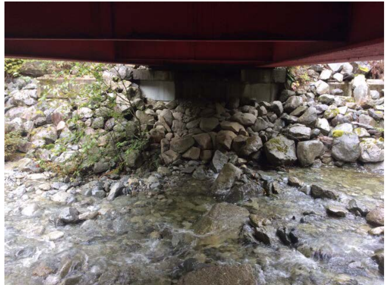
Right Bank Abutment when facing downstream
