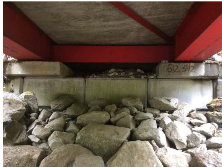
Left Bank Abutment when facing downstream
